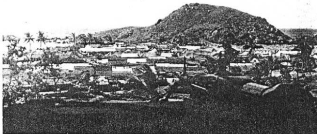
REBUILDING BEGINS—An American machinegun provides additional protection for the hamlet of Son Tra. To the right is the area burned down by the Viet Cong in their recent attack on the village, where rebuilding efforts will be concentrated. The refugees have been living in tents scattered throughout the village. (Photo by Sp4 Bill Guerrant, Photo Editor)
