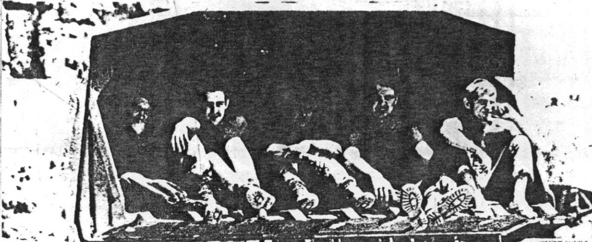
Ingenious engineers improvise by using scoop loader for balcony seats
