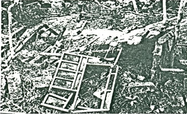
Demolished VC Position
