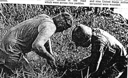
An Army combat engineer cautiously works with an ARVN engineer as they attempt to disarm a booby trap placed in the path of progress on the Mo Duc Road, 39 miles south of Chu Lai. Americans and Vietnamese worked hand-in-hand to complete the project, even on this delicate task.
